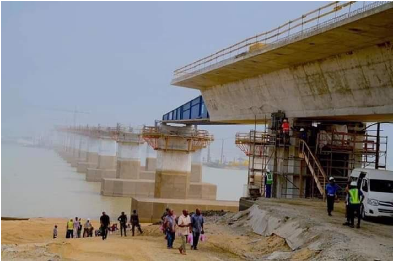
Figure 2: Muhammadu Buhari bridge
